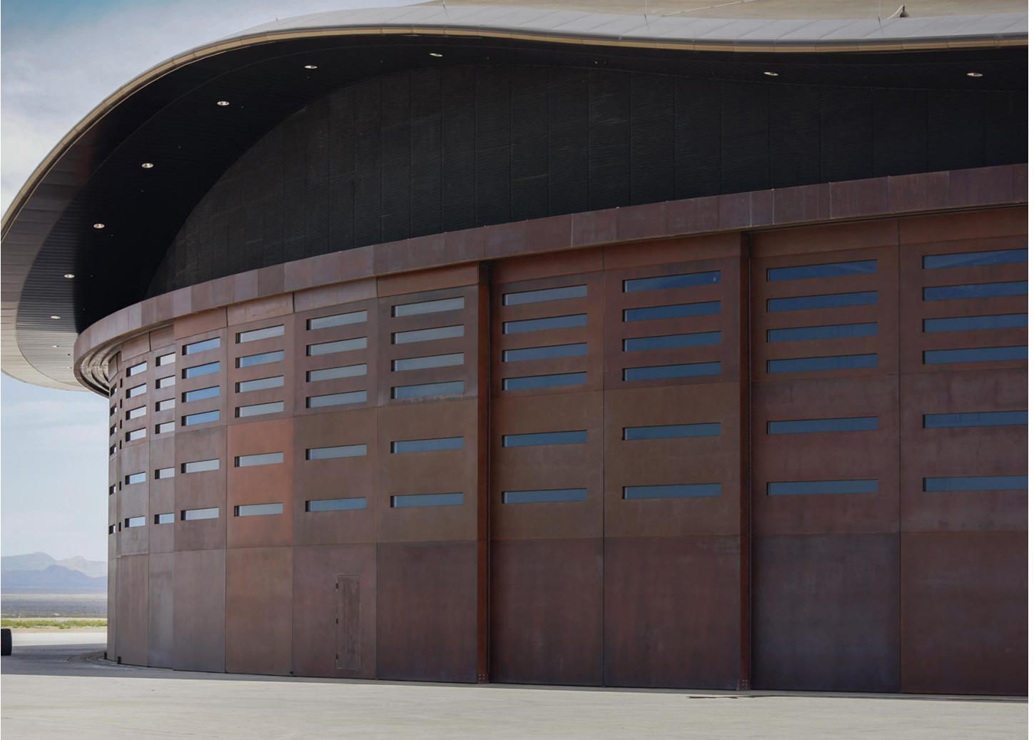
Plate Panels in Solanum™ Steel on Spaceport America in New Mexico.
