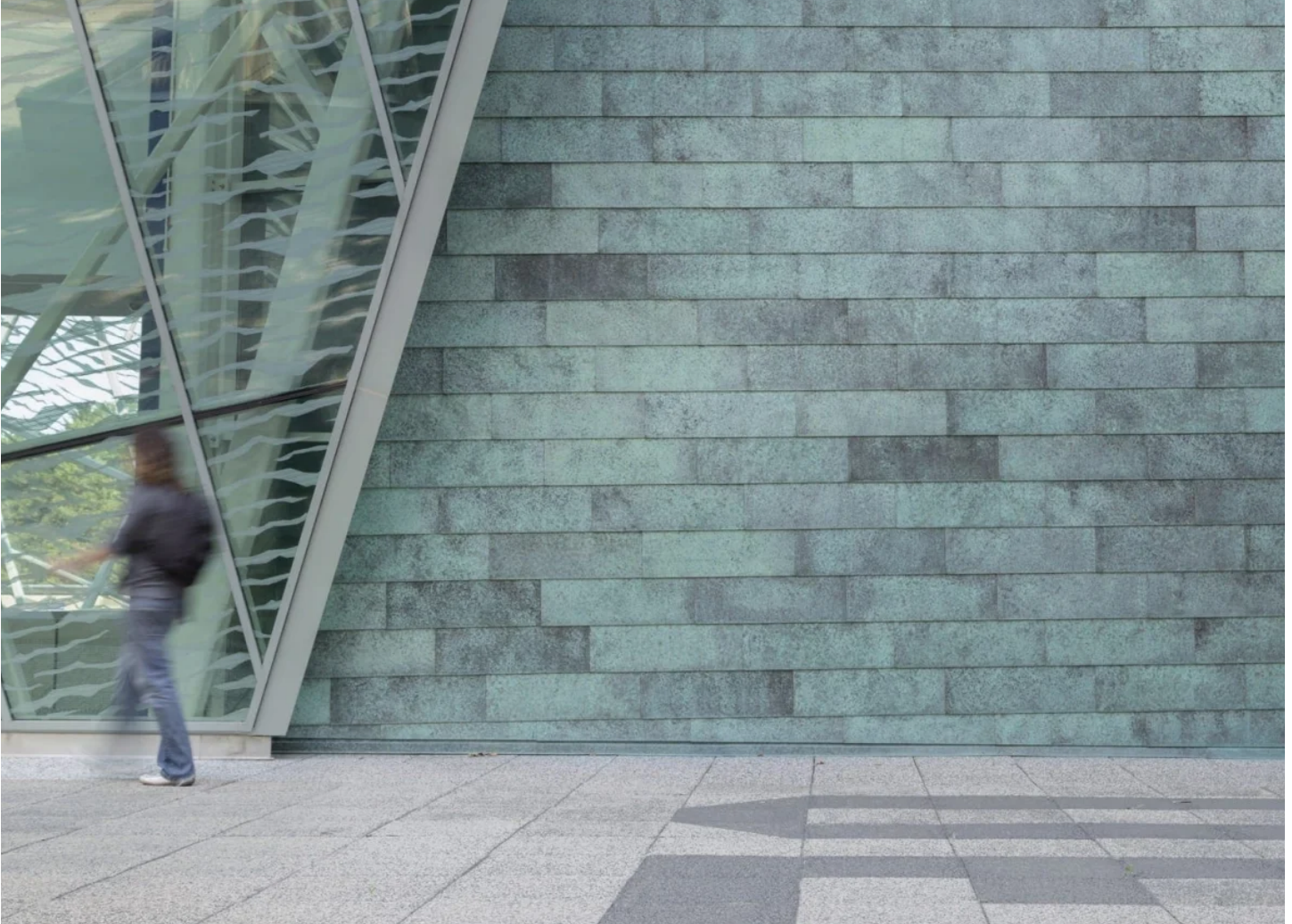
Flat Seam panels in Star Blue™Copper at SUNY New Paltz Student Union Building.
