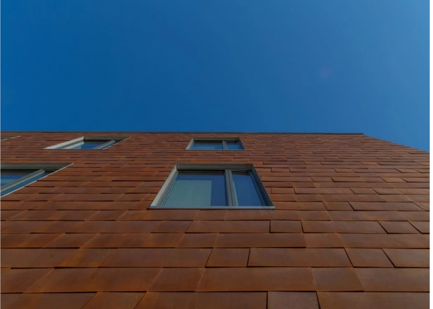
Flat Lap in Solanum™ clad the Brown University Applied Math building.
