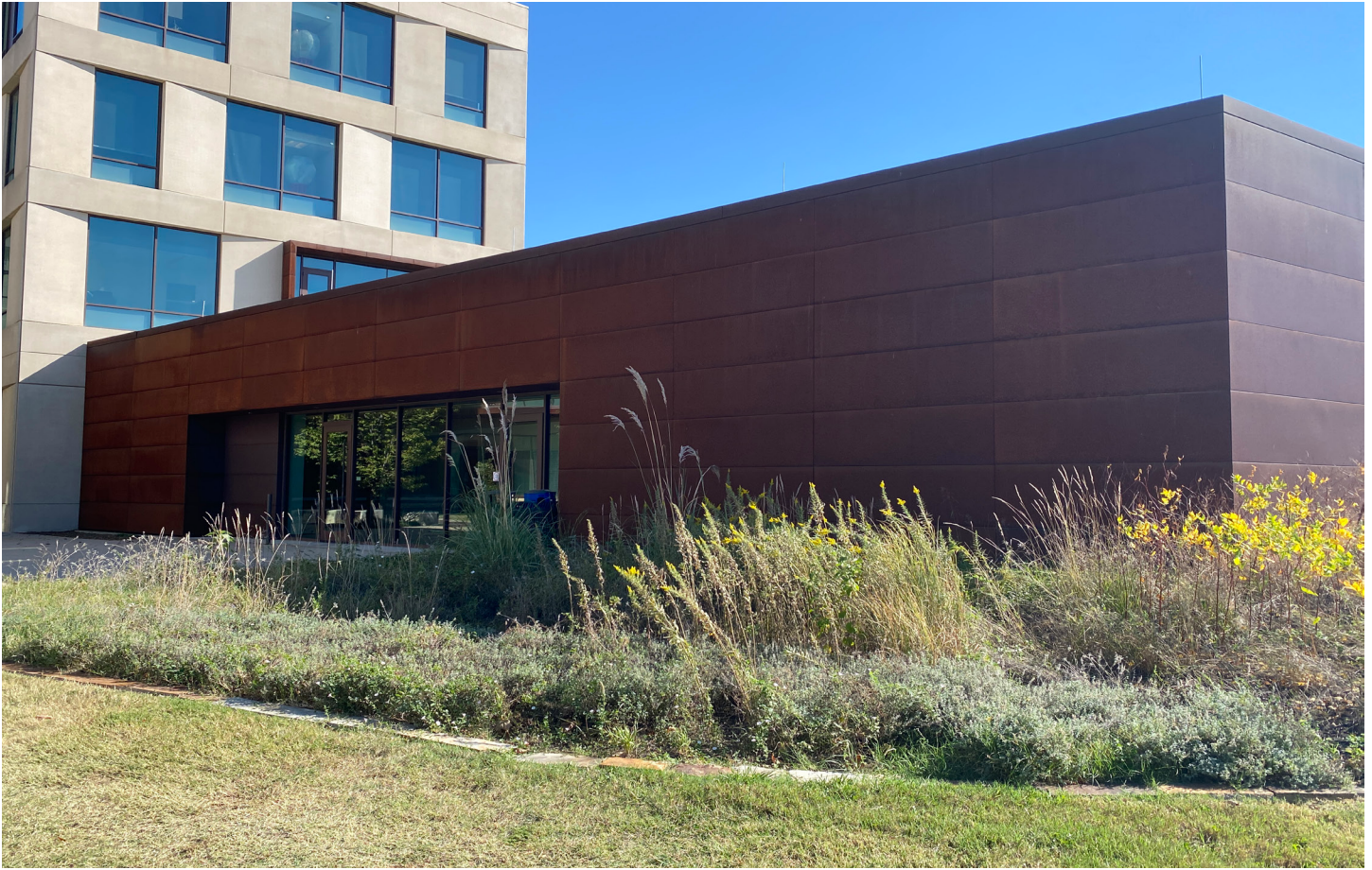
LockAlign™ panels in Solanum™ Preweathered Steel at Kansas University Capitol Federal Hall Building.
